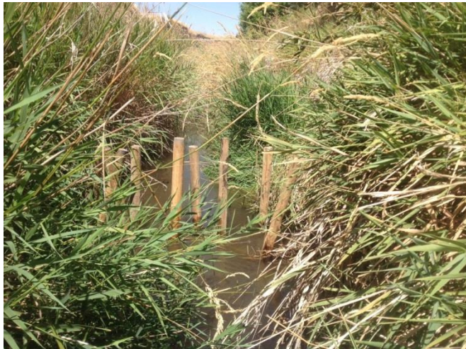
Complex 3. BDA trial # 5. Primary dam. Looking upstream prior to adding willow.
