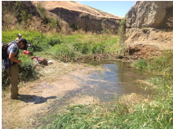
Complex 1. BDA trial # 2. Primary dam. Note large gravel deposit on river right. Looking downstream.
