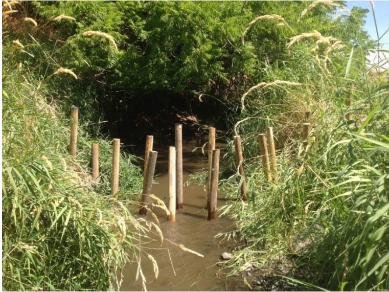
Complex 4. BDA trial # 6. Secondary dam. Looking upstream.
