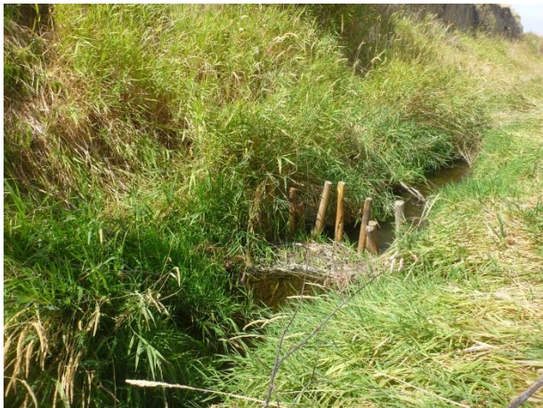
Complex 2. BDA # 3. Reinforcement of the start of a natural dam.
