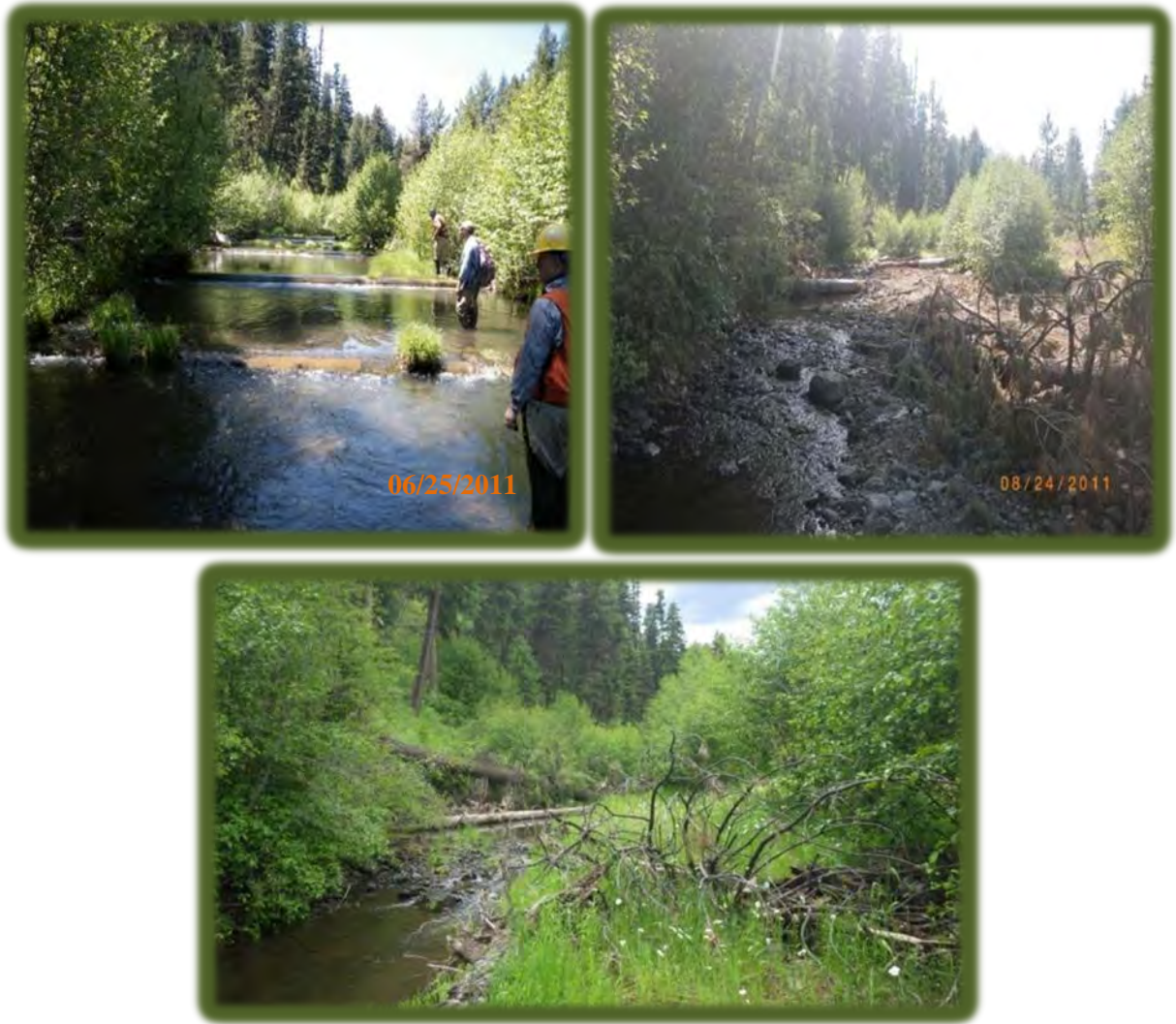
Figure 49: Log Weir Removal from Reach 4 of Camp Creek before (top left), immediately after (top right), and 3 years later (bottom)
