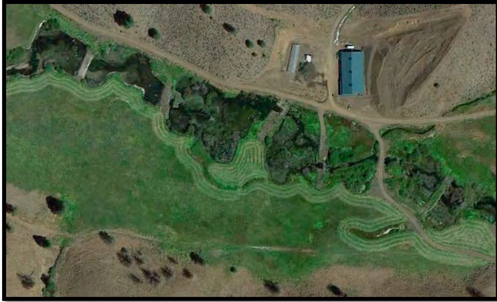
Figure 32: Examples of rock and gravel dams that are called “artificial beaver dams” in Oregon House Bill 3217, which would exempt these structures from normal environmental review by designating this area as a pilot project. These instream structures look similar to road crossings and are substantially different from beaver dams. It is thought that these structures were placed in an incised ephemeral stream that lacked fish, but there has been no onsite verification, fish passage over gravel dams is a concern, as is the potential loss of riparian vegetation as a result of flooding. This example is from the Silvies Valley Ranch in eastern Oregon. (From Google Earth; GPS coordinates: 44.052364 - 119.004789).
