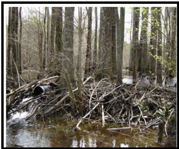
Figure 40: Flexible pond levelers with cylindrical wire cages on the upstream pipe end. Clockwise from upper left (a) and (b) are examples during the construction phase, while (c) is an example just after completion but before dam repair. (b) is a downstream view of a pond leveler after beaver have repaired the dam. Photographs from Boyle (2006).
