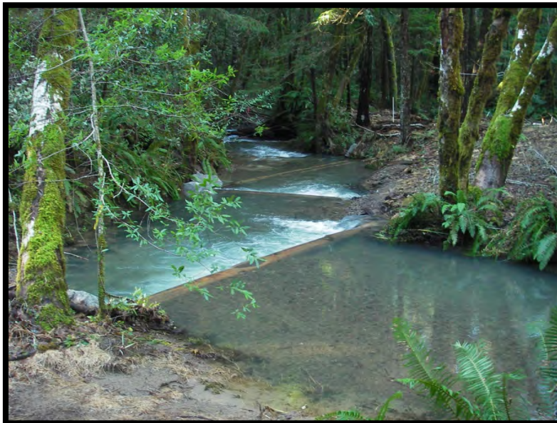
Figure 33: Log steps on the Mattole River, California, designed to raise water tables and create pool habitat for threatened coho salmon. (From McKee, unpublished).
