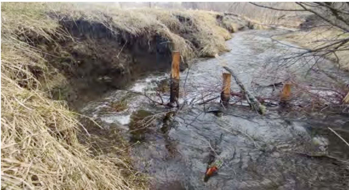
Figure 83: Breach of BDA 1 showing water flowing around the structure, eroding the left bank. This BDA is still functioning as grade control through water impoundment upstream as well as facilitating the widening of the incision trench. Notice the development of an inset flood plain directly downstream along the right bank
