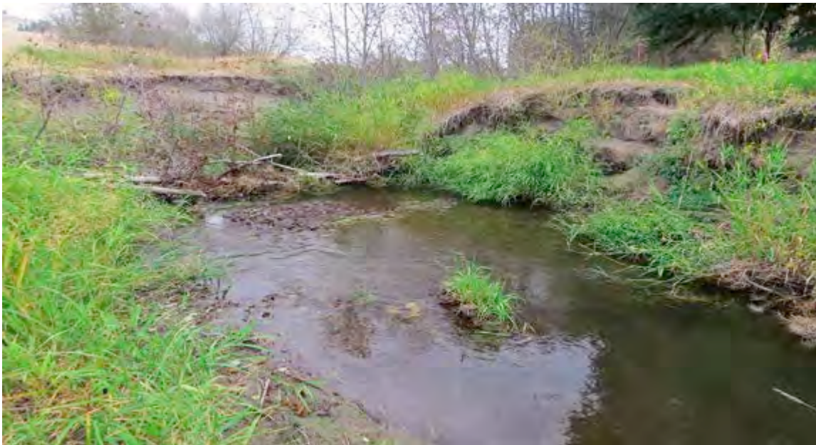
Figure 81: Before installation of a BDA and placement of LWD (see figure 82)
