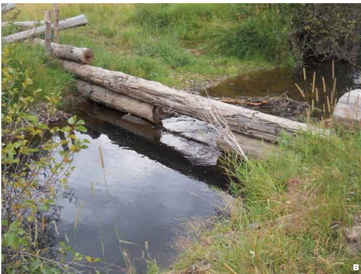
Figure 5. Two types of flow-choke structures were built: (a) with a simple contracted weir and (b) with a combined orifice and weir. Both structures impound water during high flow and are strong enough to withstand ice jams. Photo credits: Paul DeVries and Angelo Vitale.
