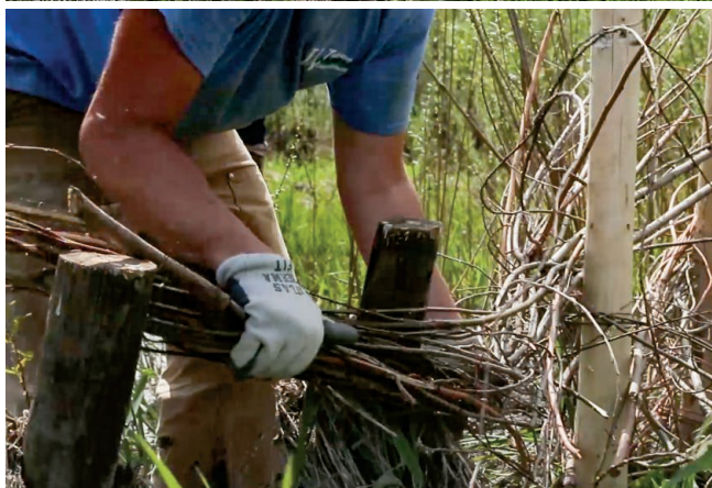
On Oregon's Bridge Creek, researchers create an artificial beaver dam by pounding logs into the stream bed (top), then weaving a lattice of sticks (bottom).
