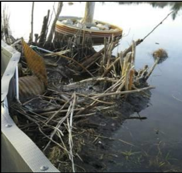
Photo 14: Side-view of dam set-up where beavers used sticks and mud to close the gap between exclusionary fence and the diversionary dam.
