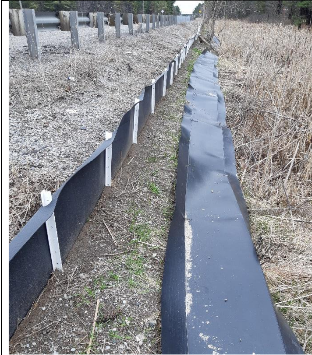
Photo 49: Viewing exclusion fence (Animex) from inside with larger stronger posts attached through the top lip of the fence 26-April-2019; no maintenance required after installation in October 2018.
