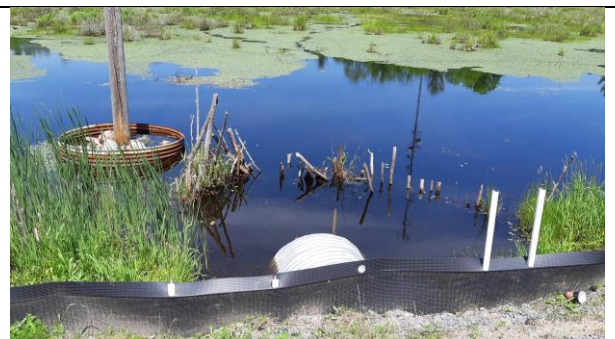
Photo 42: Exclusion fencing pulled 1 metre above north main culvert on higher ground
