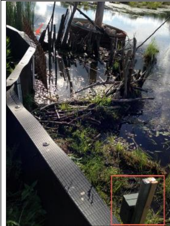
Photo 19: Camera (red box) at east side of culvert facing east side of diversionary dam. Red arrow indicates placement of second camera.
