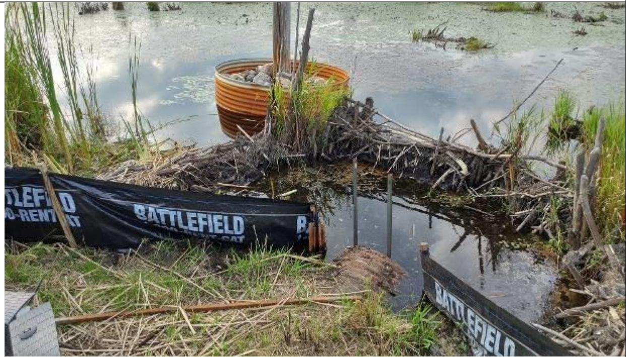
Photo 28: Silt fencing used to guide turtles to culvert on 12-Aug-2017.
