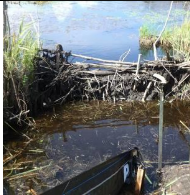
Photo 31: Secured diversionary dam on 12-Aug-2017.
