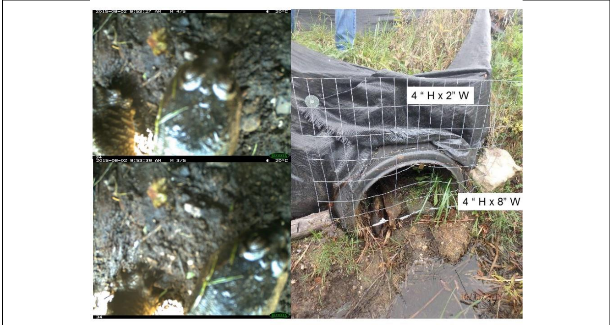
Photo 3. Exclusionary wire screen on the east side of the drainage culvert entrance with larger mesh size at the culvert opening (right) and pictures of Snapping Turtle trying to enter culvert but turning around (left).
