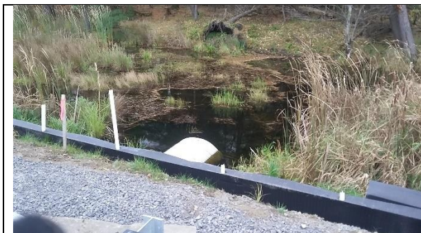
Photo 41: Exclusion fencing pulled 1 metre above south main culvert on higher ground
