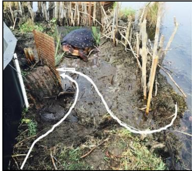
Photo 13: Gap between dam and exclusion fence where a turtle (pasted into photo) could access the culvert, later beavers closed this gap with sticks and mud (Photo 14).
