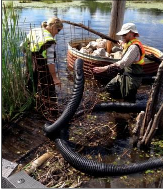
Photo 17: Implementation of cage with pipe into wetland.
