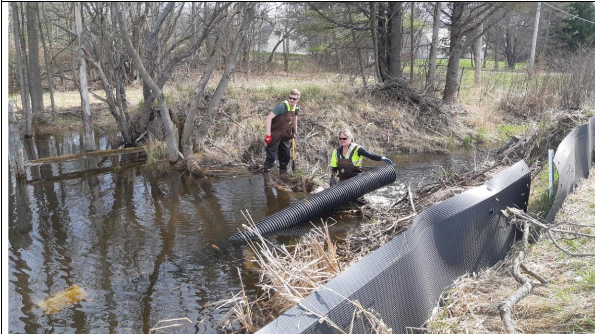
Photo 38: Placing the pipe into the beaver dam.
