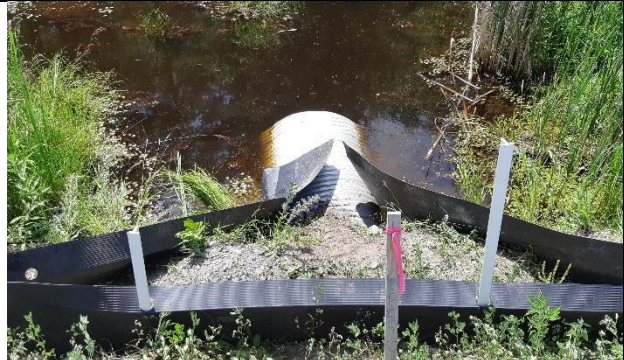
Photo 44: Guide-wall fencing extending from fence to south main entrance on 08-Jul-19
