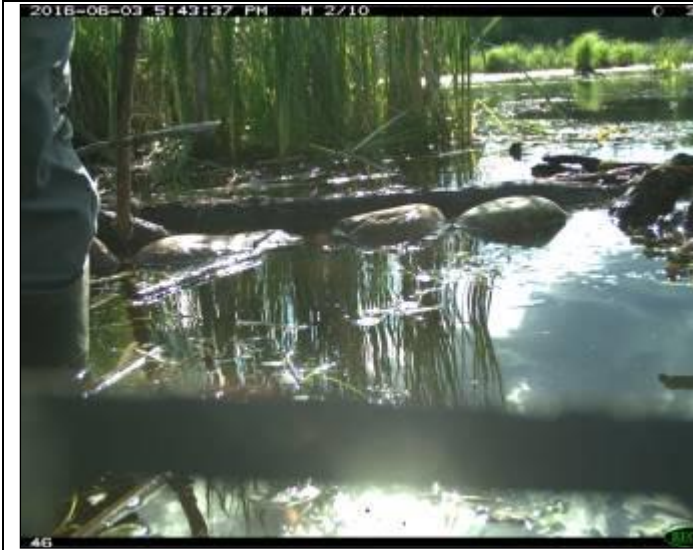
Photo 21: Initial set-up of Reconyx cameras, view of gap between diversionary dam and culvert on west side on 3-Jun-2016.
