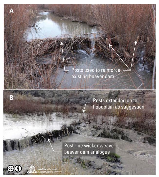
Figure 18 – Reinforced natural beaver dam (top) and post-line wicker weave BDA built in Bridge Creek (bottom).
