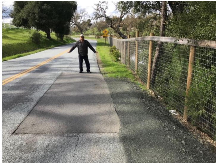
Figure G-10. Study case demonstrating size and erosive impact of a former bank den by the Spanish Lakes neighborhood in Templeton, San Luis Obispo County. The county filled in the den and rebuilt the road after it collapsed recently, due to the beaver activity.
