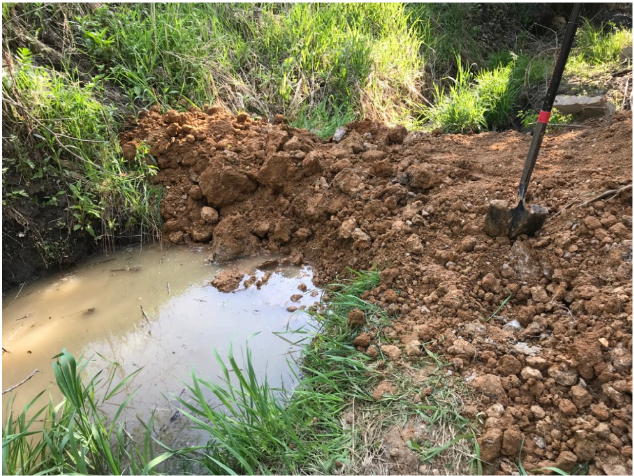
Figure 7: Clay Berm Under Construction
