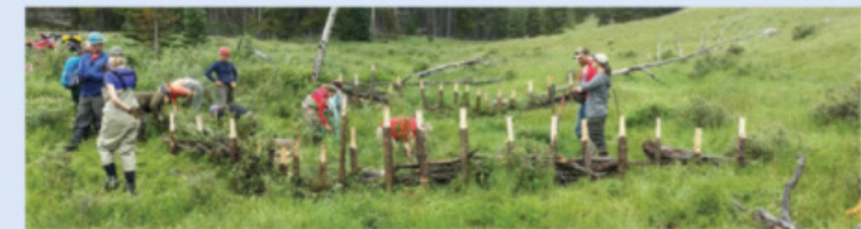
Game and Fish employees build a beaver dam analog, which simulates the function of a beaver dam. These structures help to store water and can make the area more appealing to beavers and other wildlife. (WGFD photo)
