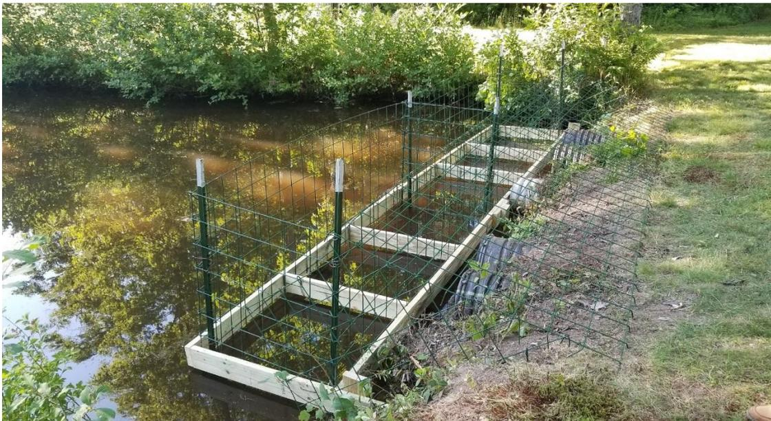
Culvert fencing installed at a homeowner's pond in Bow, NH
