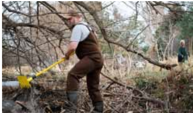
Chris Bachman of the Lands Council installed a pipe and cage system on Linda Jovanovich's land.
