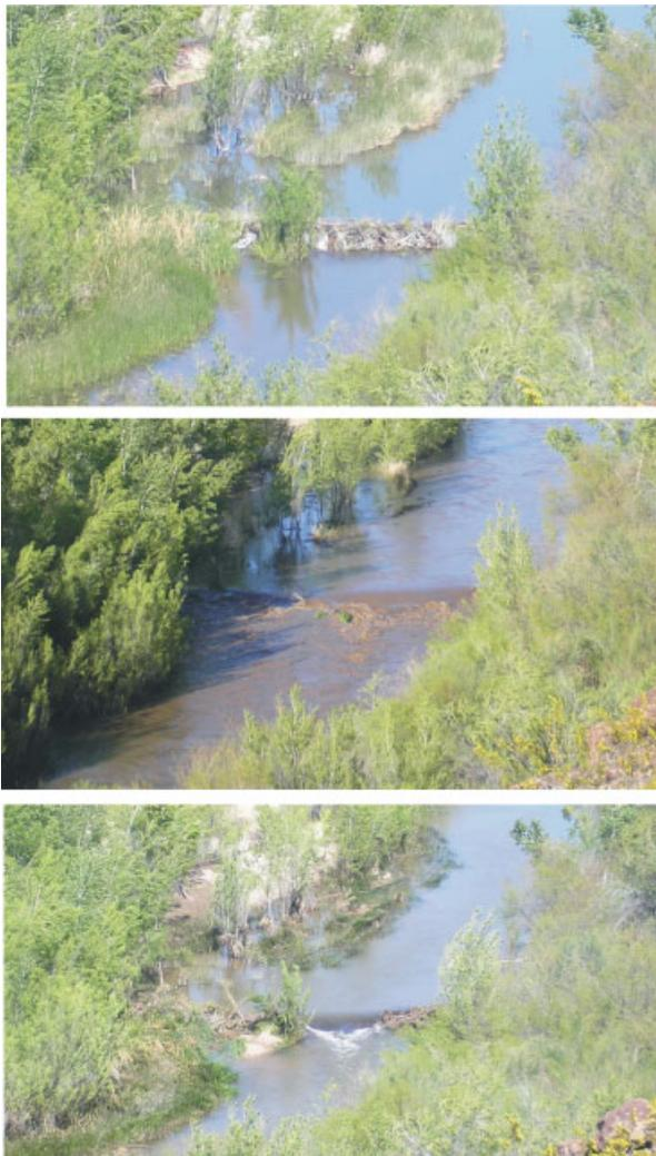
Figure 9. Repeat photographs showing Dam PC-G a few hours prior to arrival of the 2008 flood pulse (top panel) and being overtopped by that pulse (middle panel). The dam suffered a central 3.9-m breach (= major damage) that lowered the pond's surface elevation (bottom panel), but retained some functionality based on the 40-cm drop through the breach present  $\sim 2$  days post-flood. Photographs by Brad Cannon and Tom Liptrott, US Bureau of Land Management.
