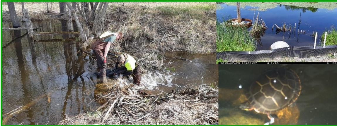
Installing a pond leveler pipe to allow water flow and prevent upstream damming at the culvert
