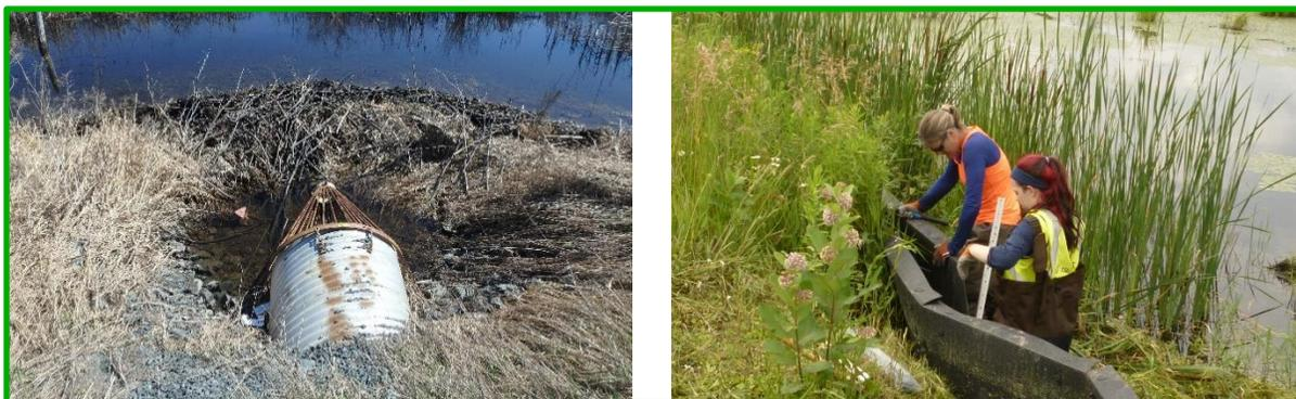
Road culvert blocked by beaver cone and dam Building wildlife exclusion fence to culvert
