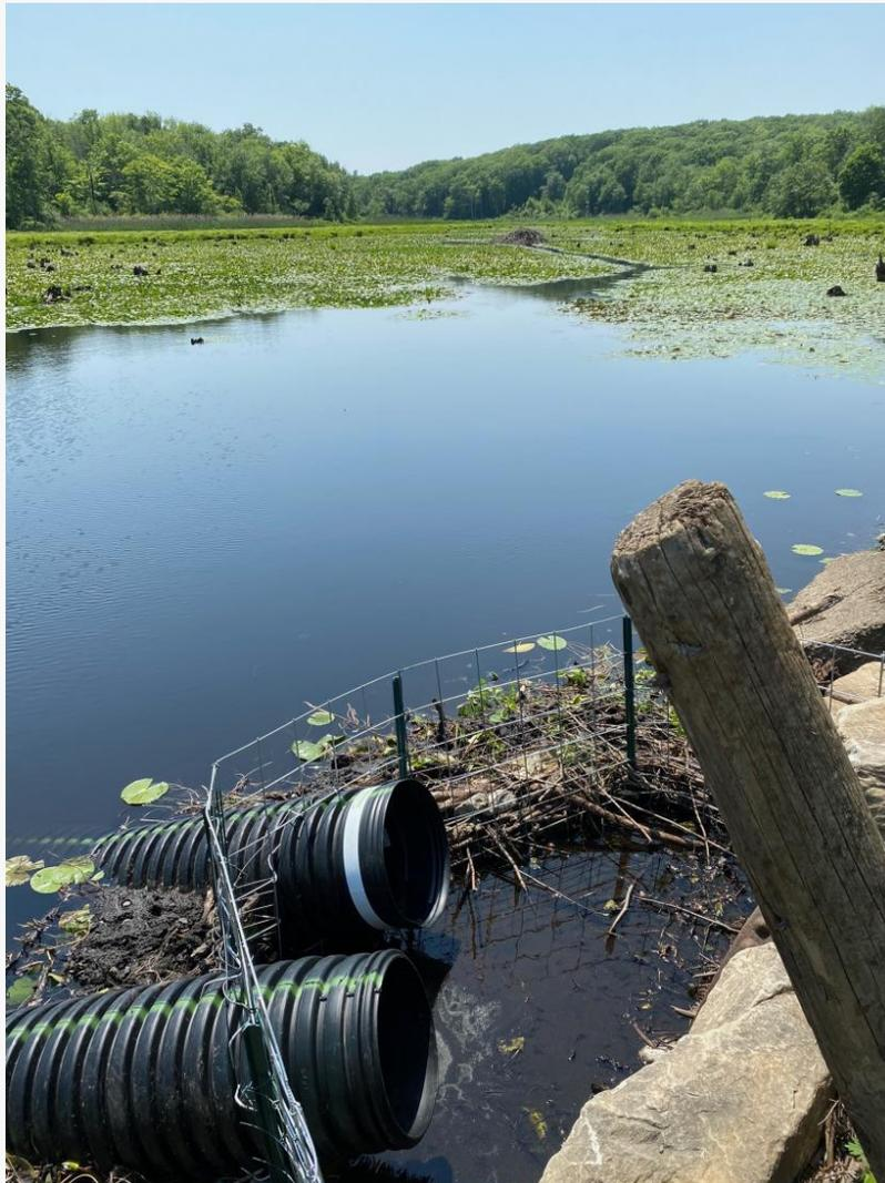
An ingenious flow system, installed in June to foil beavers, is protecting a culvert along West Woods Road #2 in Sharon, keeping the water flowing and preventing road flooding. *Photo by Leila Hawken*
