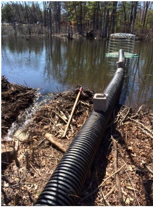
Pond Leveler Being Installed, Rangeway Rd.
