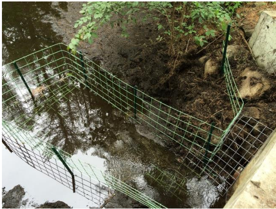
Billerica Culvert Fence w/ Wildlife Passage
